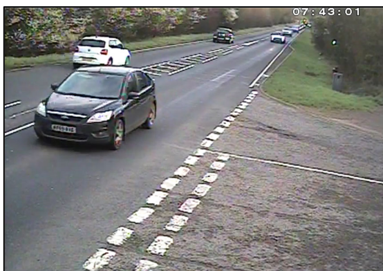
Figure 8.6: Queueing Cleared After the Road Narrowing on Burnham Road
