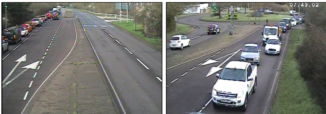
Figure 8.5: Queueing on Burnham Road Due to Narrowing From 2 lanes to 1 lane
