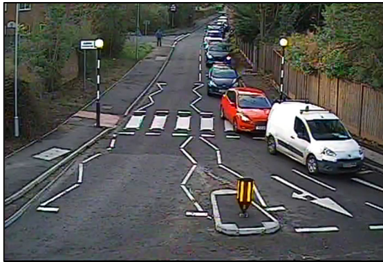
Figure 8.4: Queueing on Hullbridge Road
