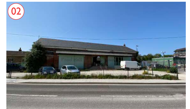
Goods Shed [c.1860] - Grade II Listed
