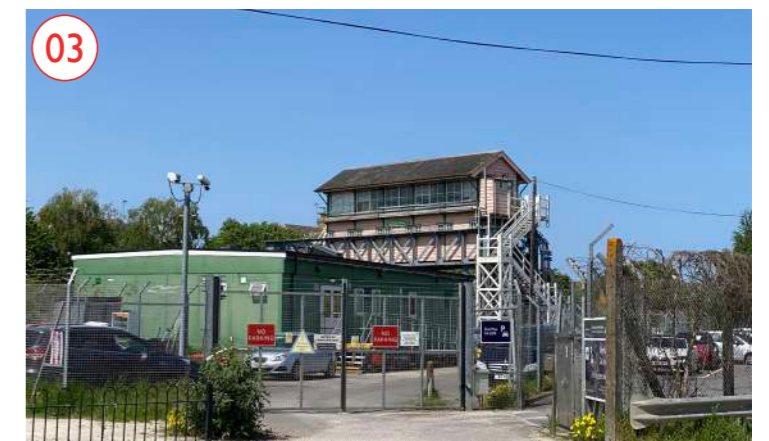
Overhead Signal Box [Late C19] - Grade II Listed
