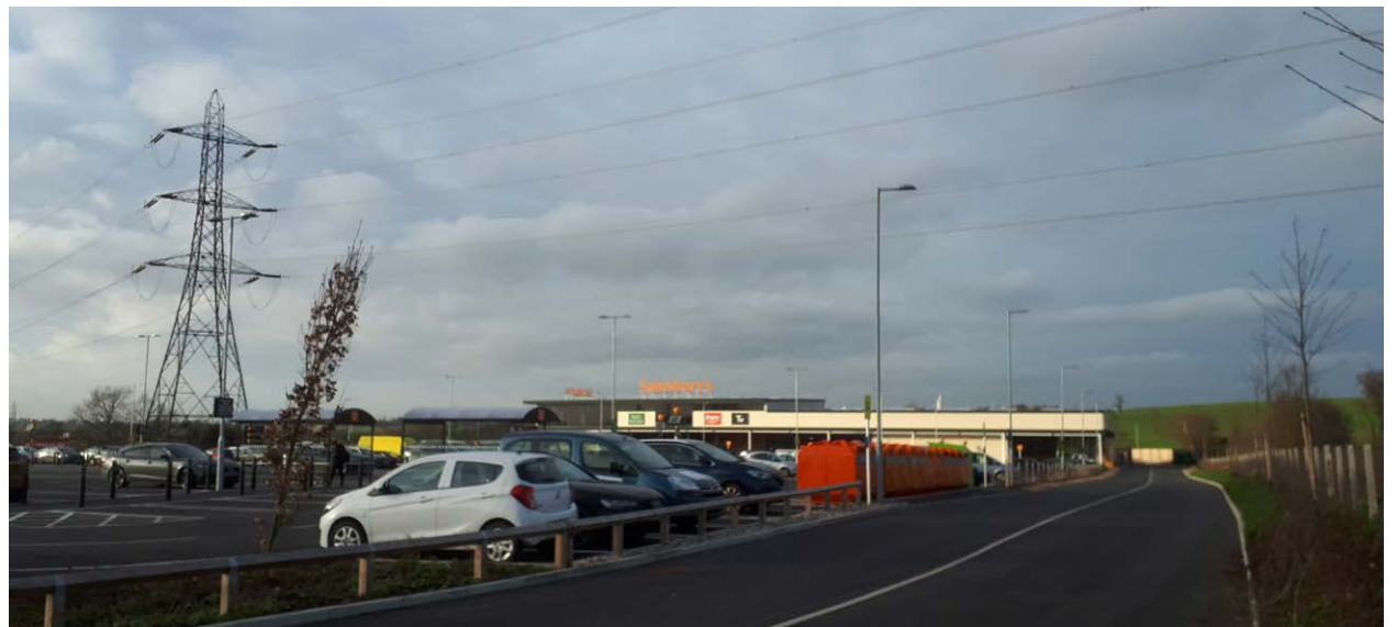
Overhead powerlines within the site
