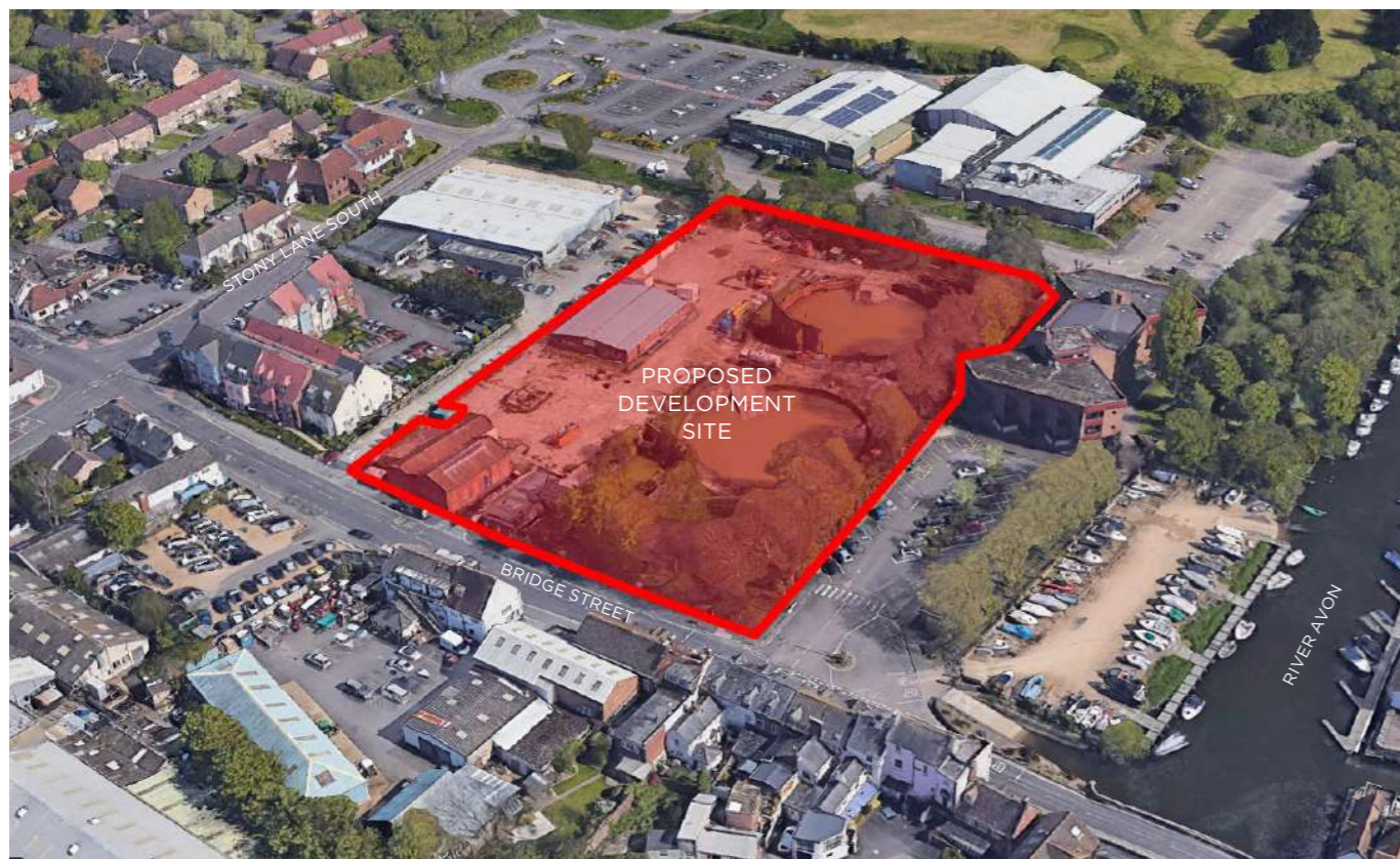
AERIAL VIEW OF DEVELOPMENT SITE LOOKING SOUTH EAST
