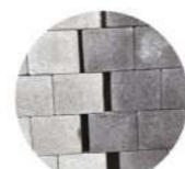
Block Paving for frontage - water ripple effect
