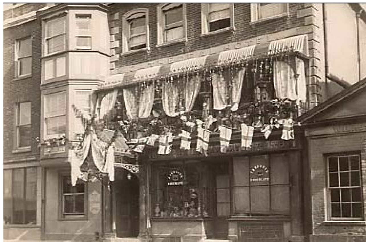
Photograph showing the original frontage
