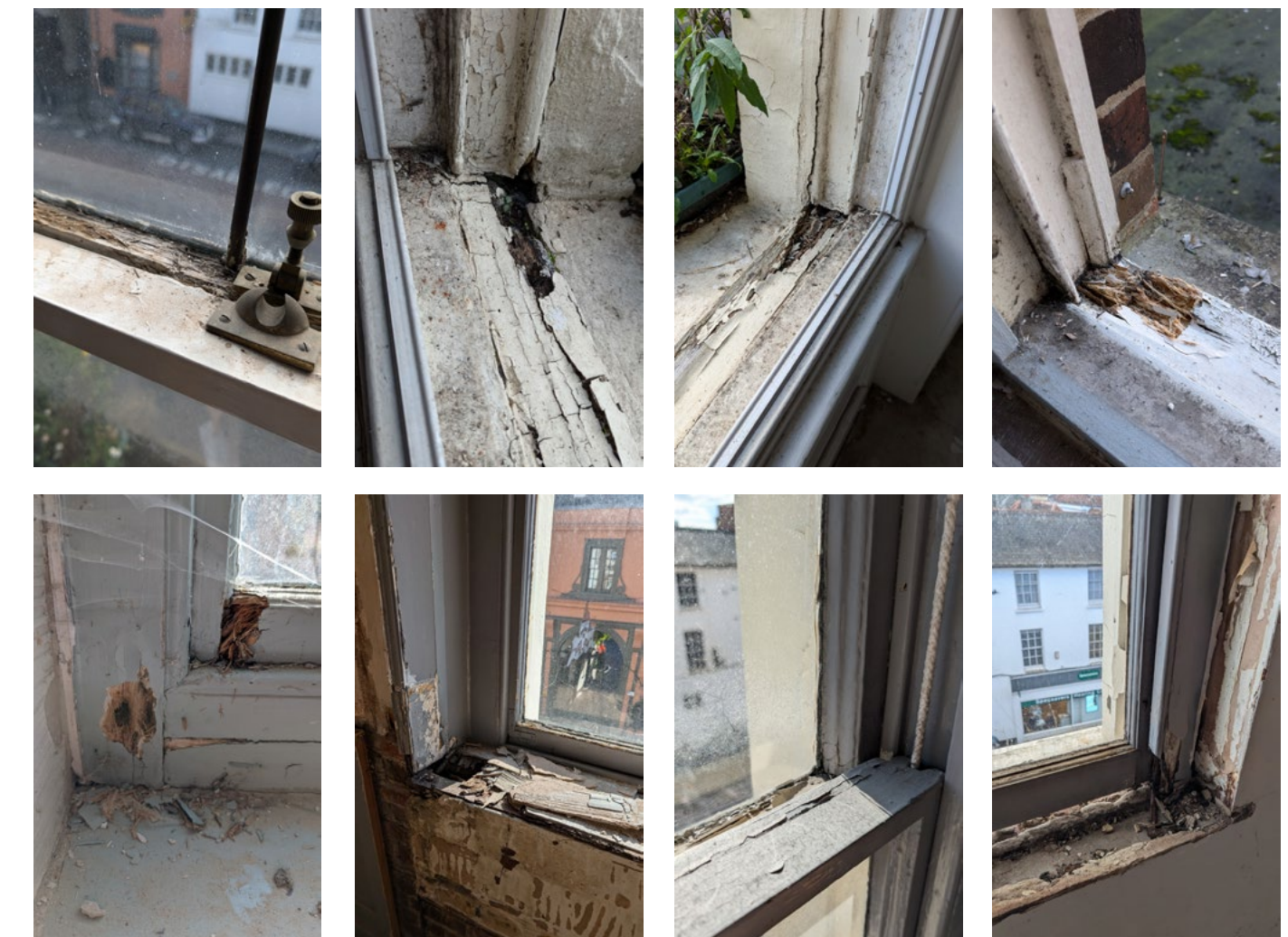
Site photographs showing the current condition of the windows
