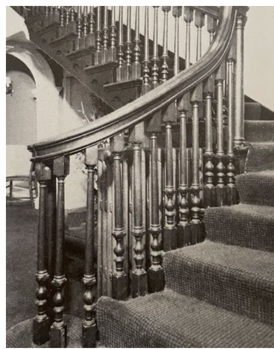
Photograph showing the original staircase
