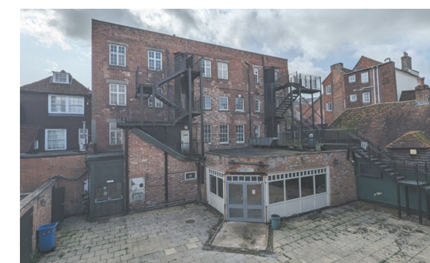
Existing Rear Courtyard
