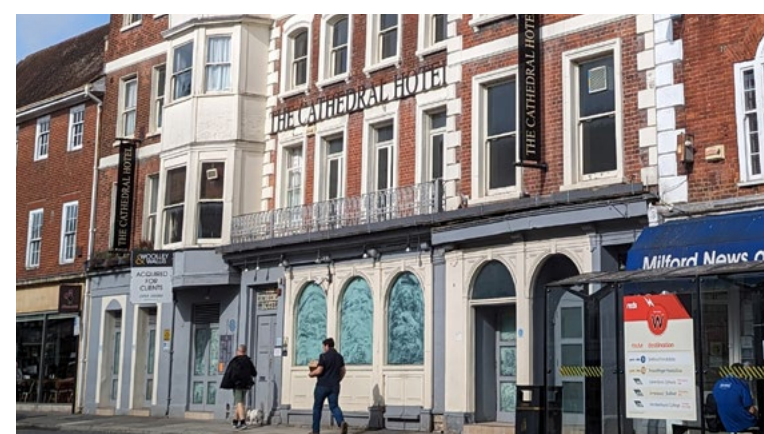
Photographs of Existing
