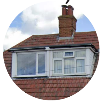
Front facing window dormers
