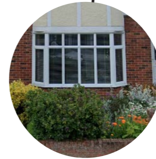
Dark red multi facing brick and white upvc windows
