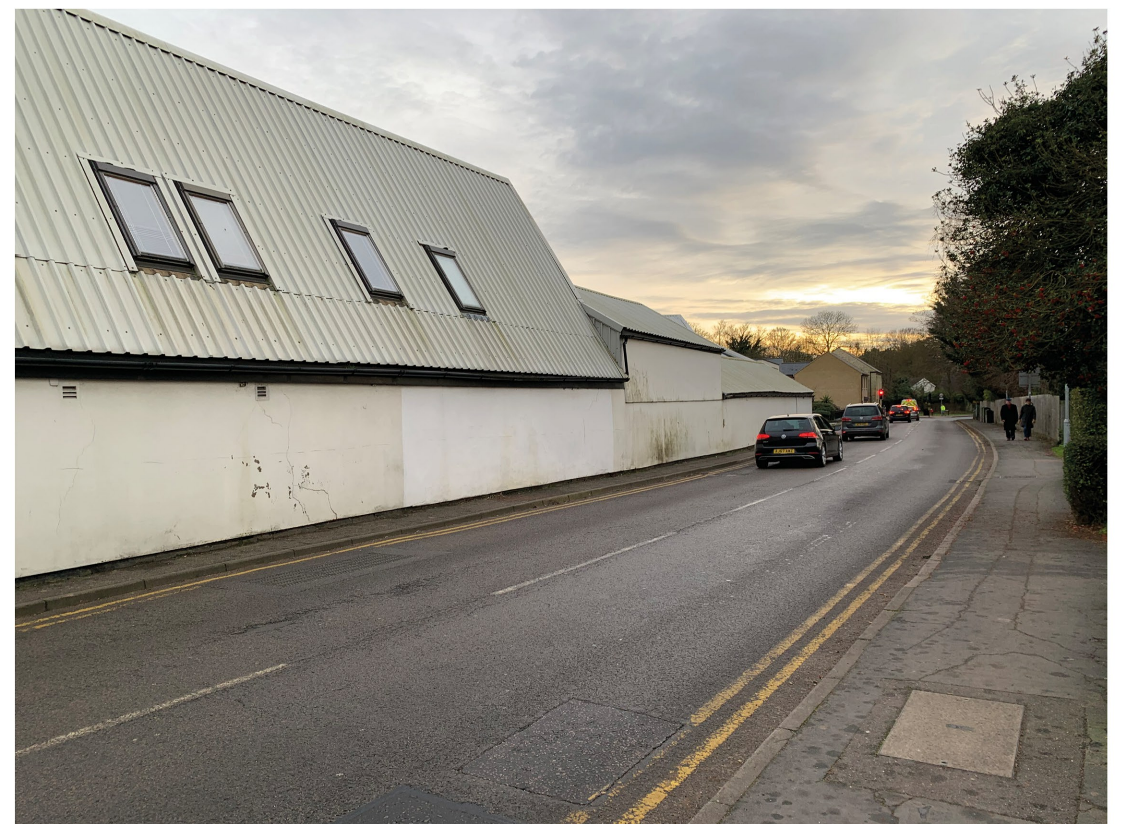
The existing building on site
