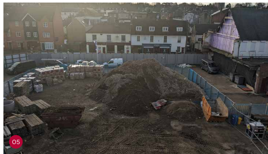
View South over site towards 28 - 36 Railway Street
