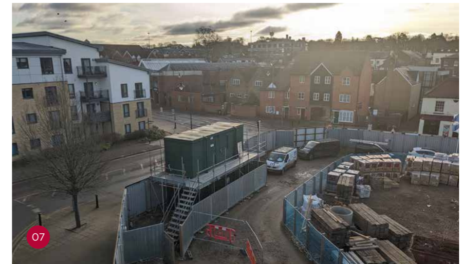
View south-east from Car Park towards Bircherley Court
