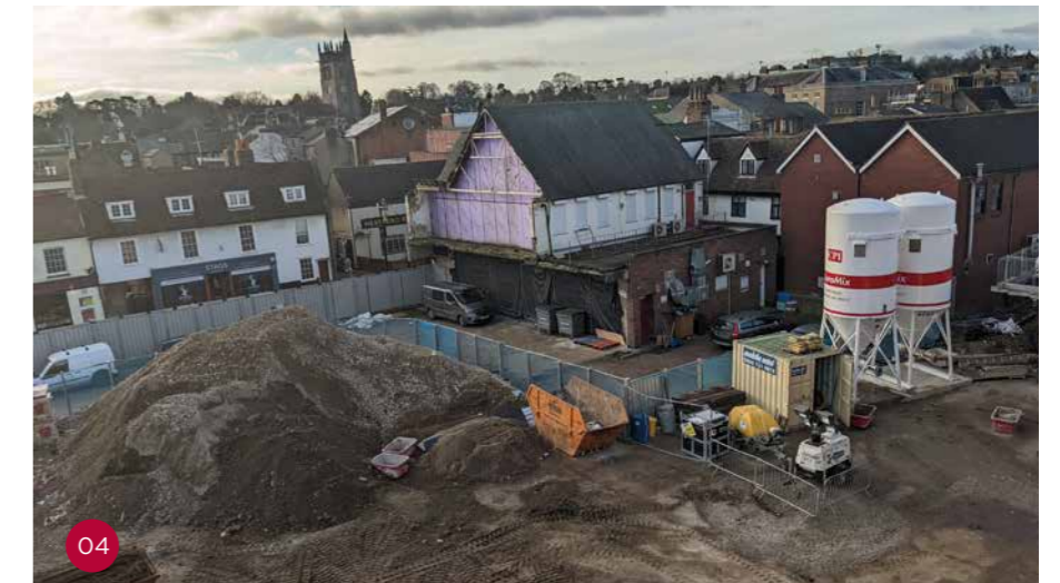
View south from Car Park towards rear of 31 and 33 Railway Street
