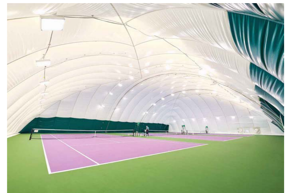
Fig. 25 Internal of typical air dome
