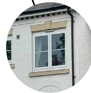
Cast stone heads and cills; white painted brickwork
