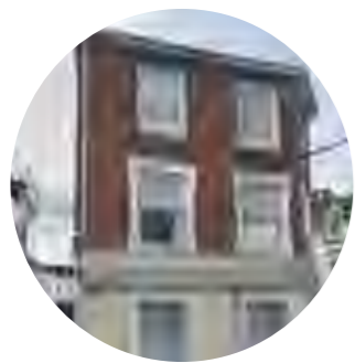
Rendered ground floor, with brick upper floors
