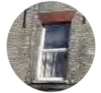
Red brickwork window heads
