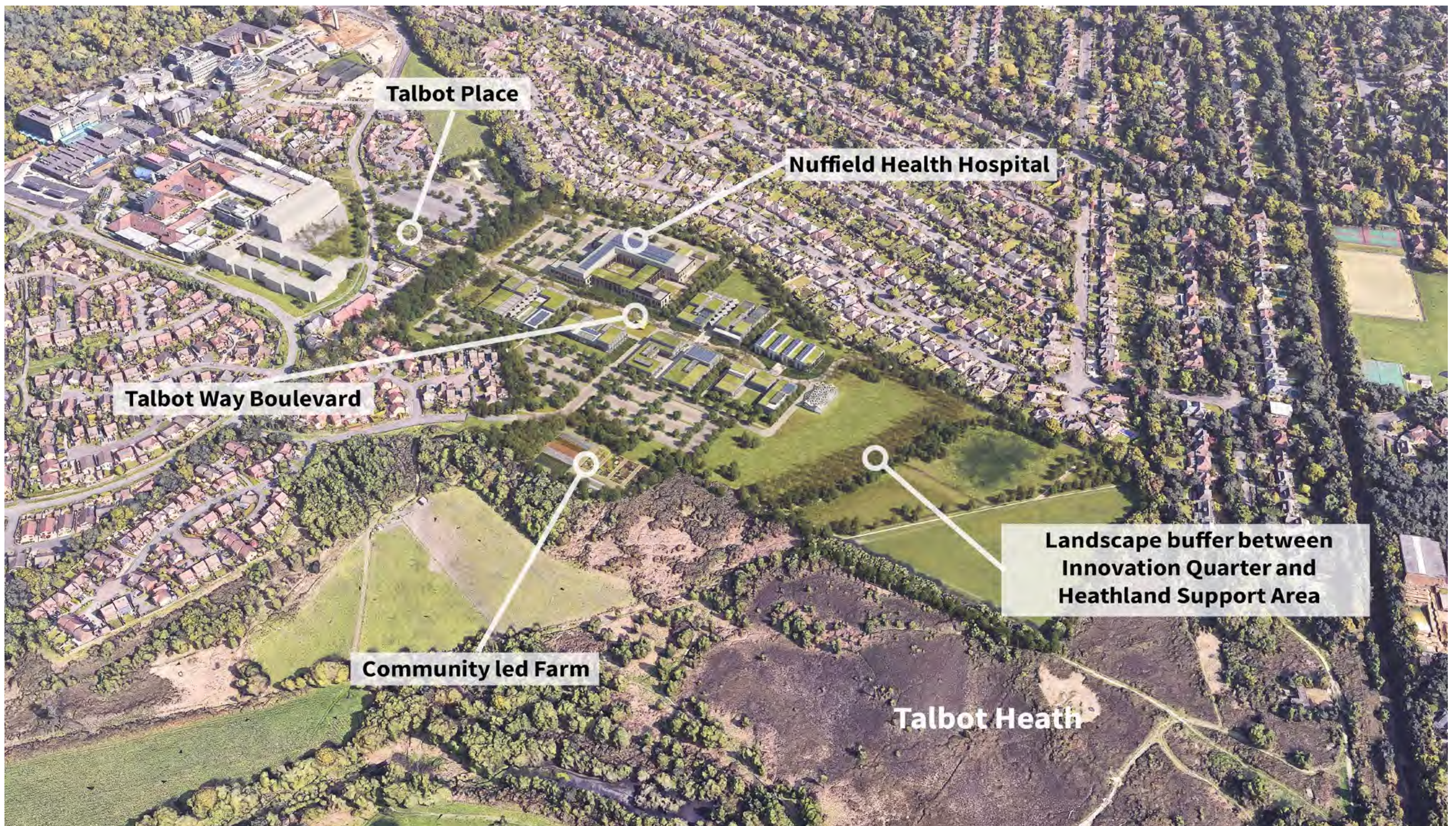
Aerial view from the south west
